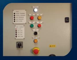
Control panel showing variable speed drive in 250 L/min increments
